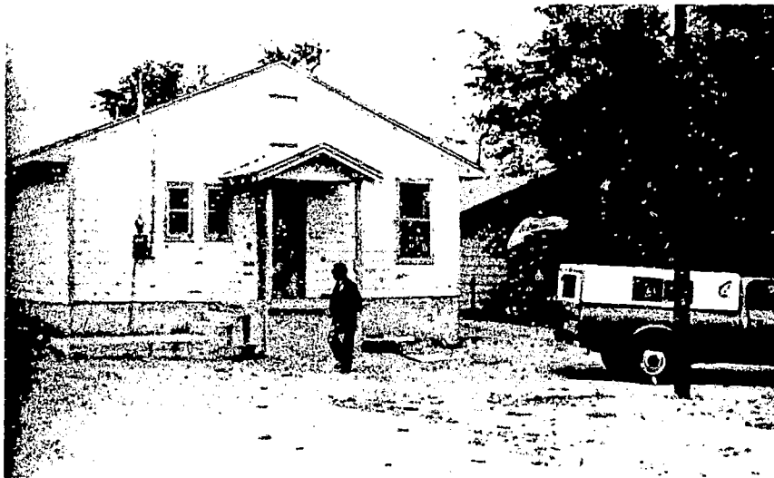
Figure C.16. Bylas Health Center Showing Approximate Site of Proposed Building Addition and Antenna Support.
