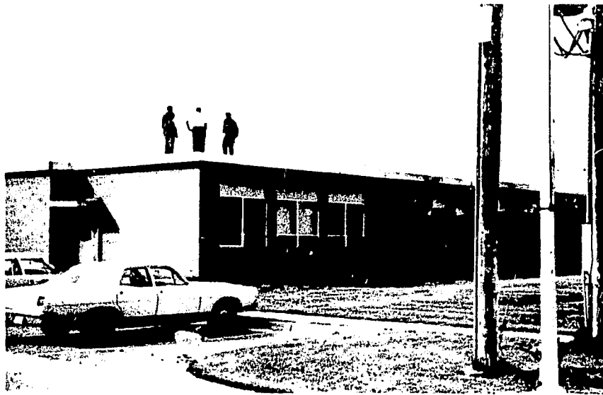
Figure C.13. San Carlos I.H.S. Hospital, Corner of Building Nearest to Teleco Equipment Room and Where Tower is to be Located.
